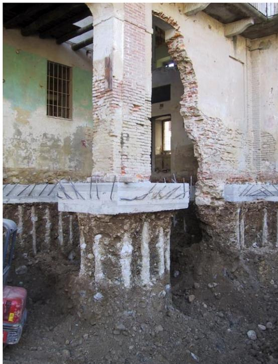
**Figura 5** - Sottomurazioni mediante micropali – Coutesy by GEOCIPO srl.
